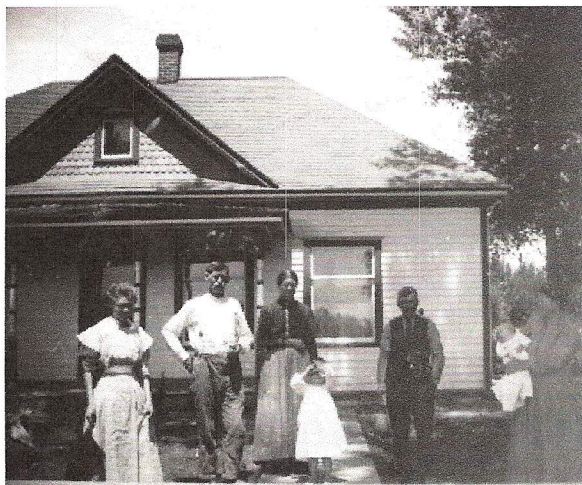
The Decker Farm at Ault, Colorado
